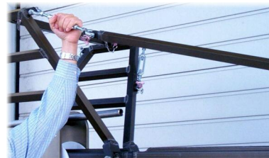
Tensioning the turnbuckle
